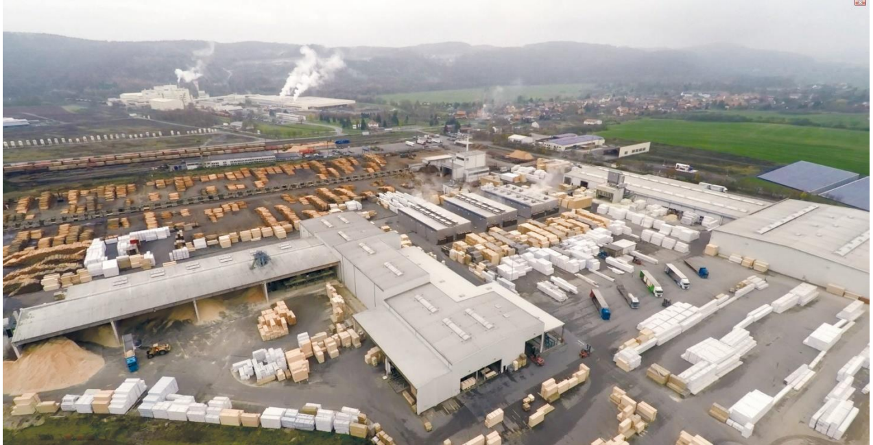
ante-holz GmbH in Rottleberode
